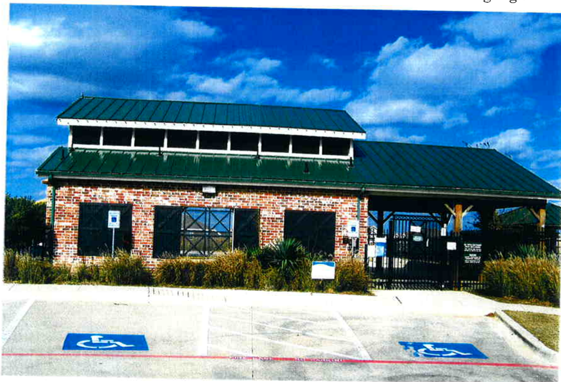
Front (Entrance) Elevation of Amenity Center Bath House Building
